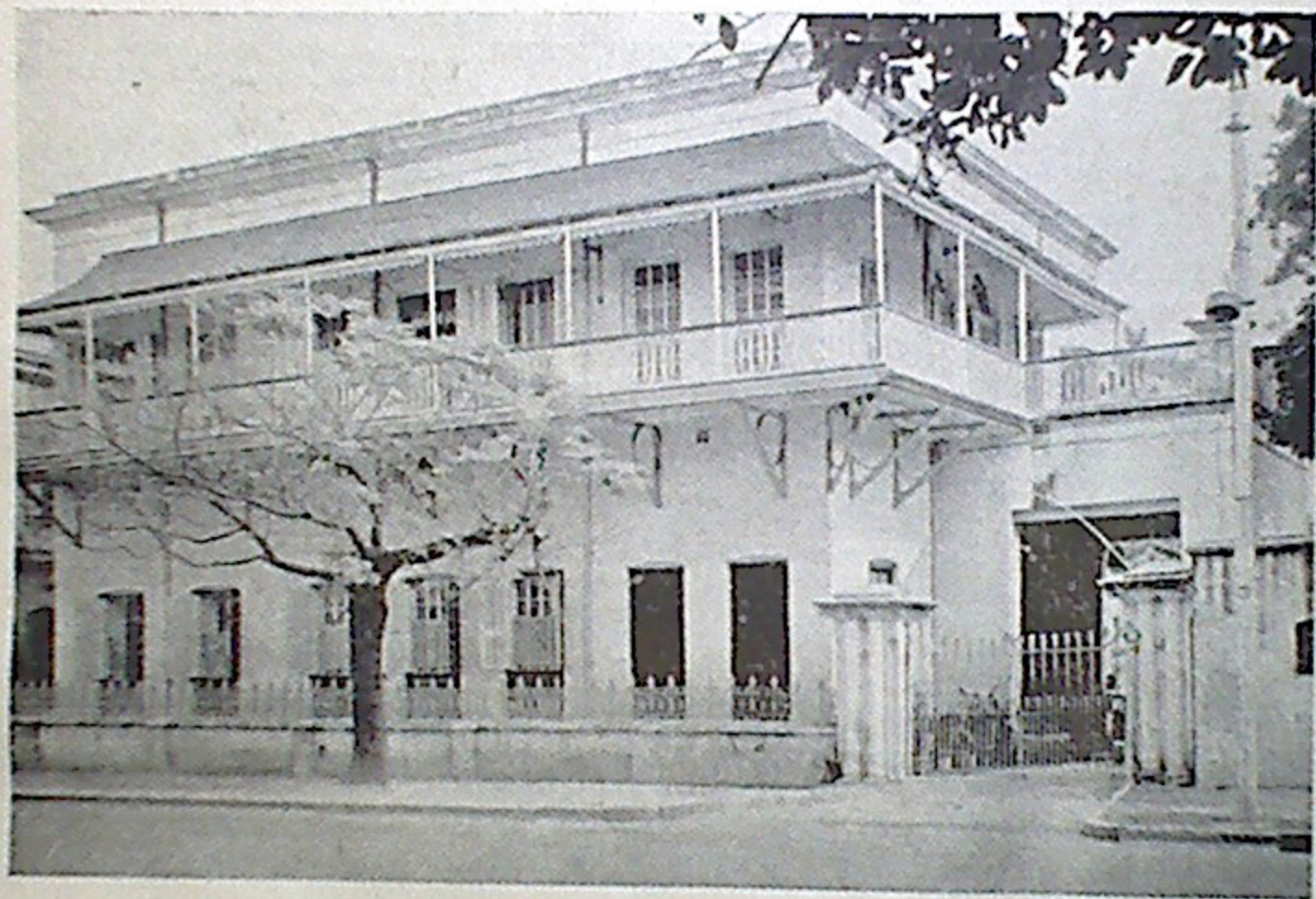
SOUTH SUBURBAN COLLEGE BUILDING 26, LANSDOWNE ROAD, CALCUTTA. ( 1916-17 )
